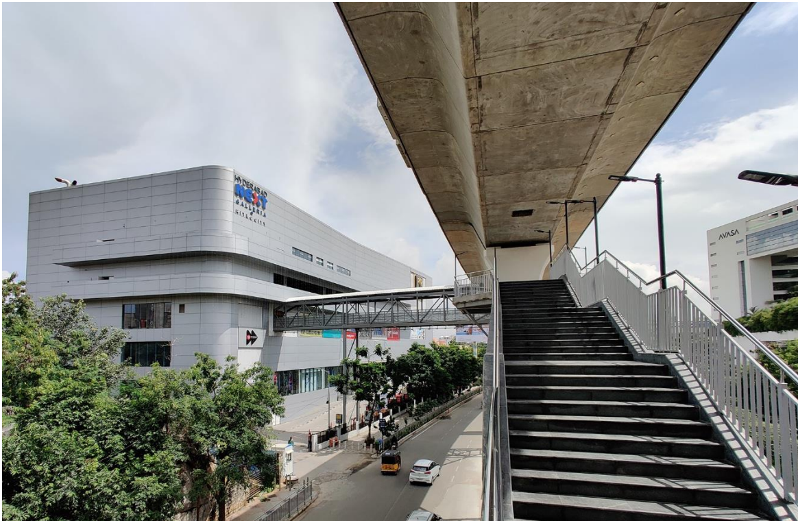
Skywalk at Hitec City Metro Station
