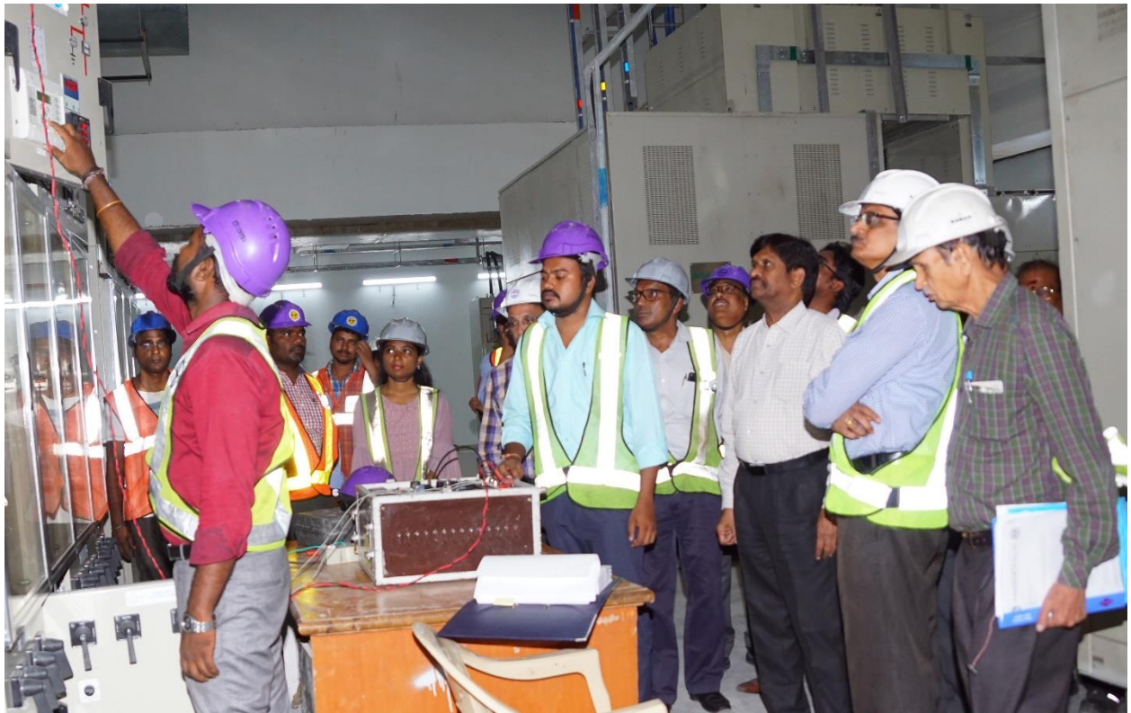
Mr. DVS Raju, CEIG along with other officials inspecting an auxiliary substation.
