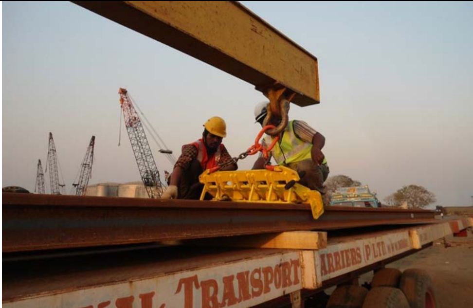
Rails being loaded on to a trailer to be transported to Hyderabad
