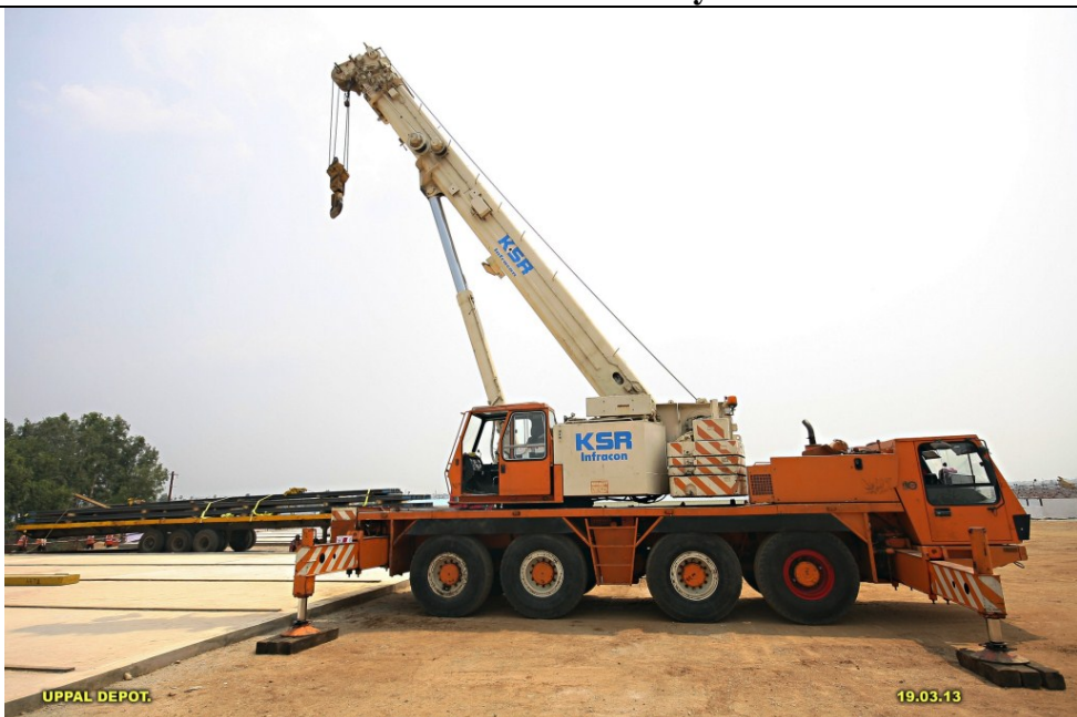
Arrival & storage of Rails in Uppal Depot, Hyderabad
